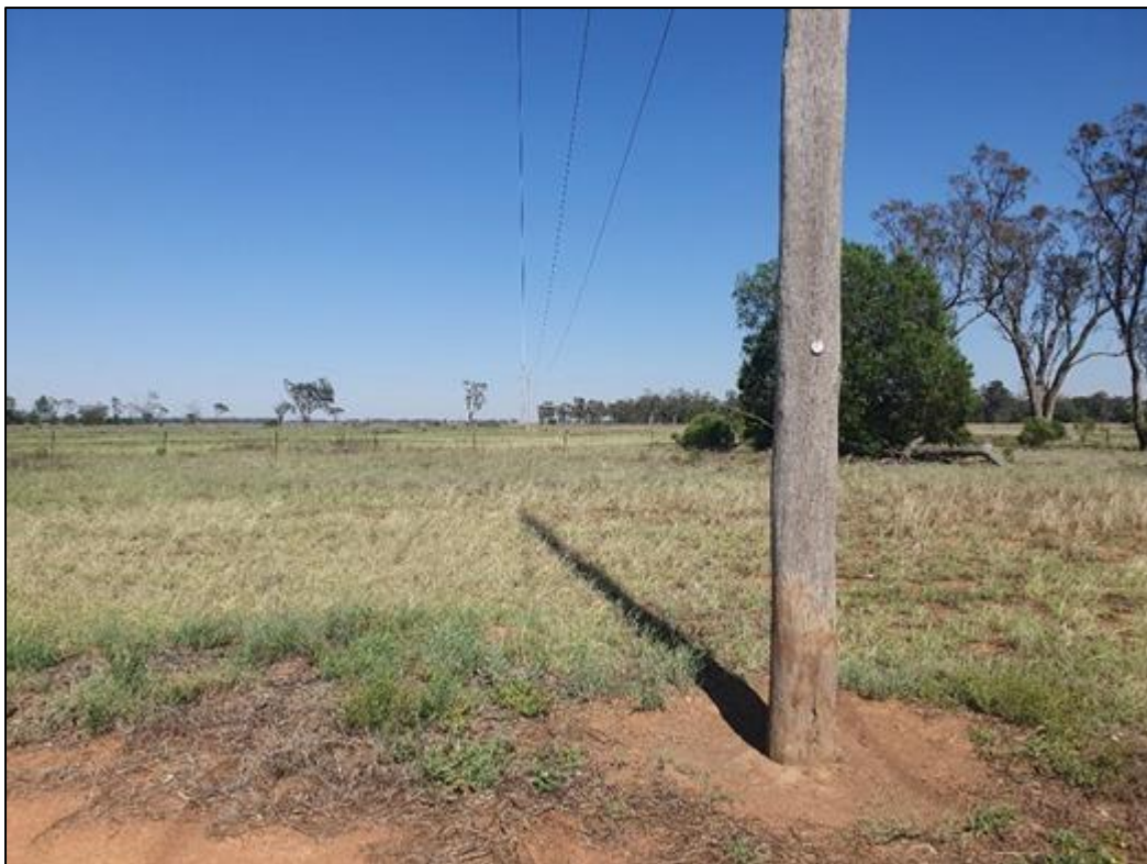
Figure 6: Site to the west
